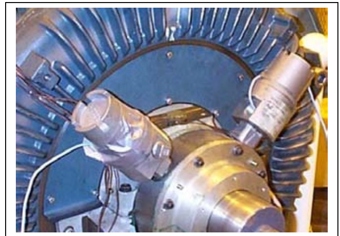
Fig. 4 - TEFC Motor with Proximity Probes Mounted 45 degrees from Vertical
